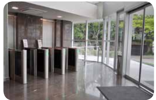
dGate installed in a commercial building in Porto Alegre, southern Brazil.
